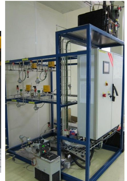
C 4 F 10 loop and plant.
